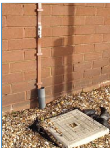
Figure 51. Typical down-conductor connectors.
